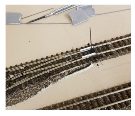
Put double-sided tape on the bottom of switch machine (trim so as not to block any of the holes).
